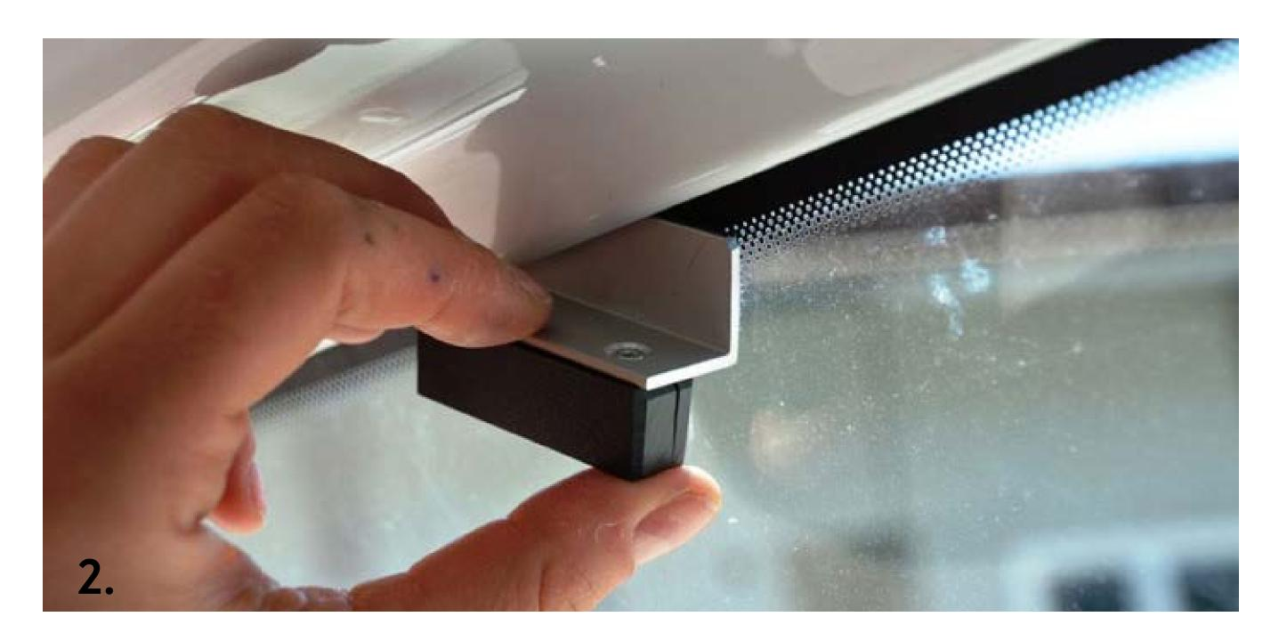
Plug the Z-angles on both sides of the window between lining and window glass (pic. 2).
